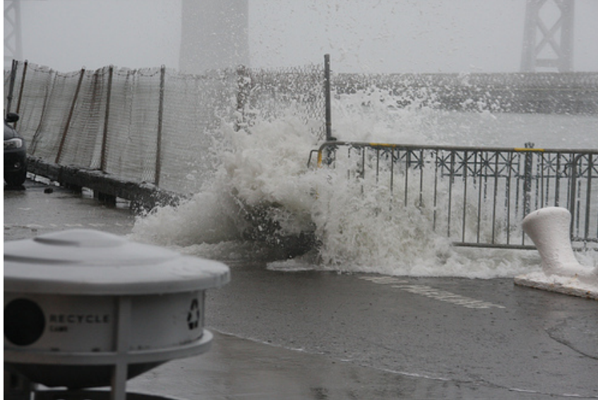
Figure 16. San Francisco's Pier 14 During the King Tide in the Winter of 2010/2011. The extremely high tide flooded sidewalks and pounded the base of the Oakland/Bay Bridge (in the background). King tides provide a glimpse of the future when sea levels are permanently higher, thus elevating regular tides, base flood elevations, and the risk of coastal erosion.
